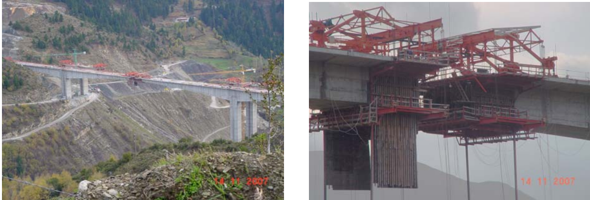
Figure 3: Views of under construction Metsovo ravine bridge, (a) General view, (b) key of central span.
